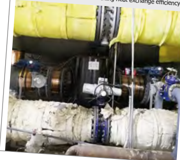
Step 2: Outdoor installation, pipe wrapped insulation cotton, X-Pro 2 unit into the protective box.
