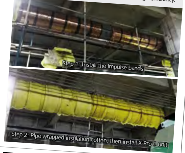
Step 2: Pipe wrapped insulation cotton, then install X-Pro 1 unit!
