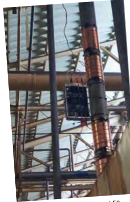
Vulcan S25 was installed around 50 meter before the induction hardening machine.
