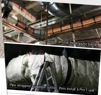
Step 2: Pipe wrapped insulation cotton, then install X-Pro 1 unit!
