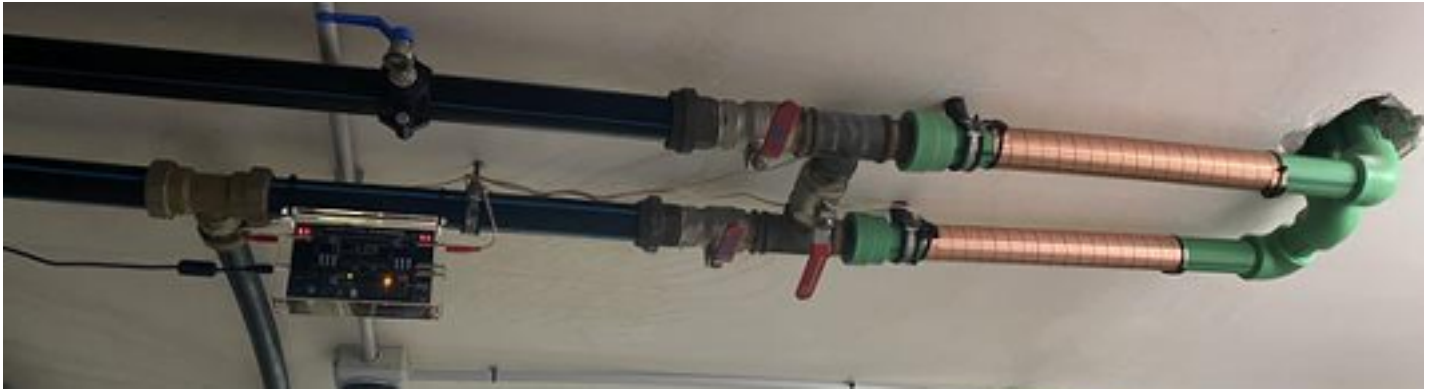
Vulcan S10 water deposit line with \varnothing 63 mm
