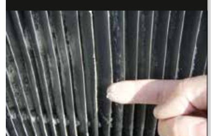
Silica could be removed by the high pressure water gun, and the remaining silica can be removed with a finger.
