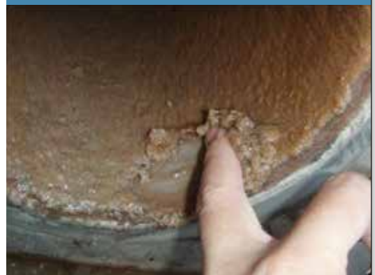
Scale becomes soft and can be easily removed with a finger.
