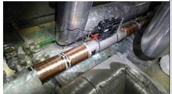
Vulcan S25 installed at Toray Industries
