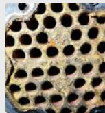
Shell and tube heat exchanger
