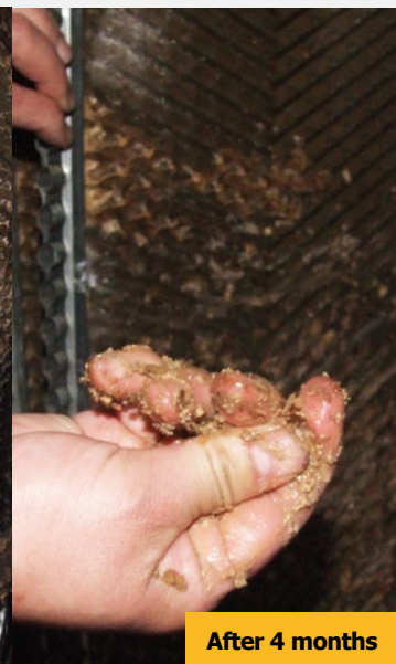
We stopped using any additional chemicals to treat the water. After installing Vulcan S250 for 4 months, the effect was very clear. Although there were still substances in the plate heat exchanger, they had been softened and could be easily removed by hands. There are no more white scales, only yellow-brown impurities left.
