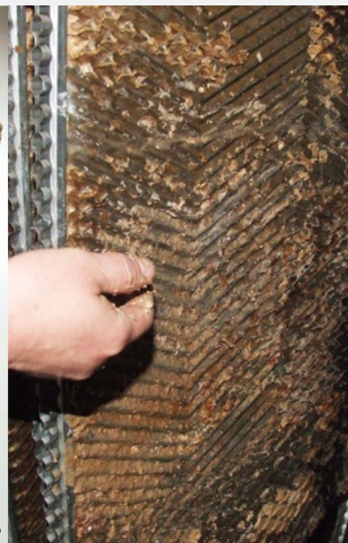
We stopped using any additional chemicals to treat the water. After installing Vulcan S250 for 4 months, the effect was very clear. Although there were still substances in the plate heat exchanger, they had been softened and could be easily removed by hands. There are no more white scales, only yellow-brown impurities left.
