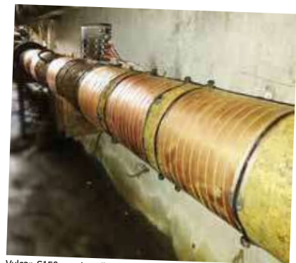
Vulcan S150 was installed on the main water pipe for the office building and the dormitory.
