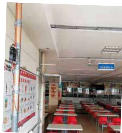
Vulcan S25 was installed to solve the scaling problems for the canteen.
