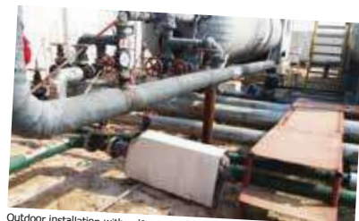
Outdoor installation with self-made cover, to protect the unit from the wind and sun.
