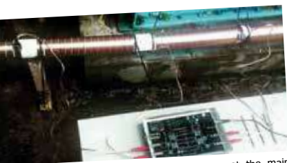
Picture 1. Vulcan installation process at the main incoming water line.
