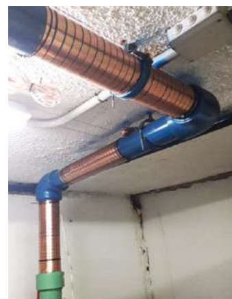
Schritt 1: Impulsbandinstallation
