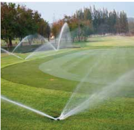
Sprinkler system on a golf course
