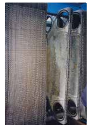
Plate heat exchanger
