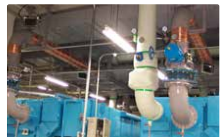
Vulcan installation in a factory
