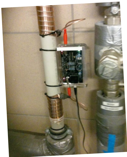
Installation des Vulcan Systems.
