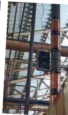
Vulcan S25 was installed around 50 meter before the induction hardening machine.
