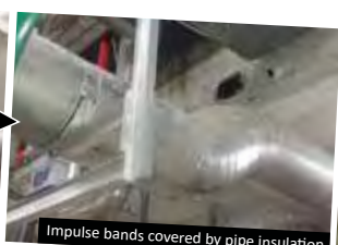
Impulse bands covered by pipe insulation
