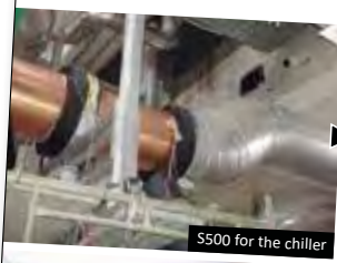
Impulse bands covered by pipe insulation
