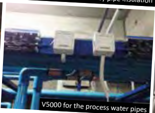
Impulse bands covered by pipe insulation
