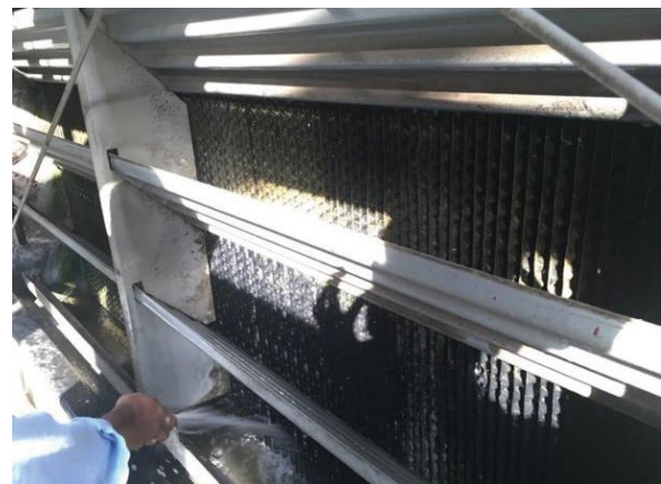
Scale and algae can be removed easily by a water gun.
