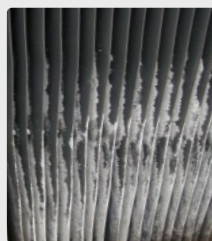
Cooling tower grids
