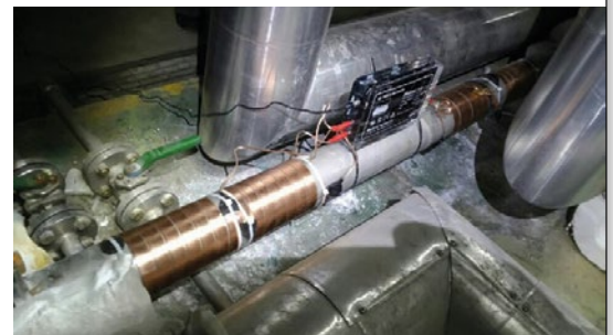
Vulcan S25 installed at Toray Industries
