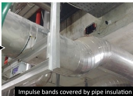
S500 for the chiller
