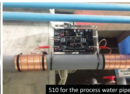
Impulse bands covered by pipe insulation
