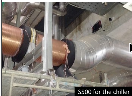
Impulse bands covered by pipe insulation
