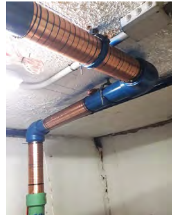
Step 1: Install the impulse bands
