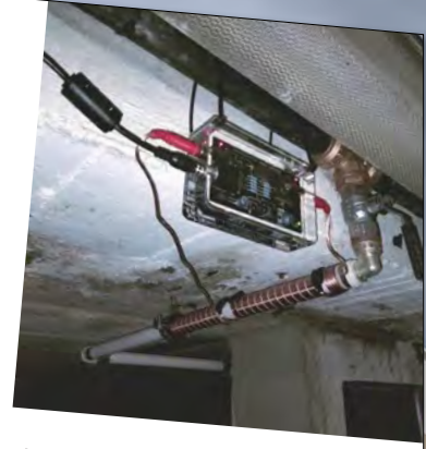
Vulcan 3000 Water deposit line with Ø 25mm
