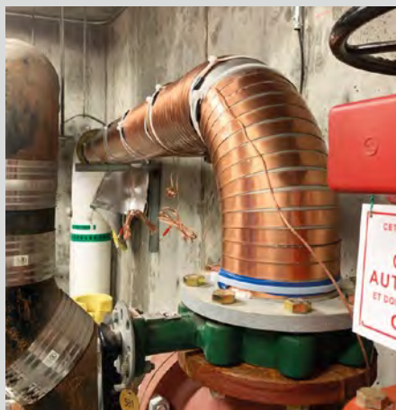
Vulcan S150 impulse bands were installed on the 8-inch water inlet.
