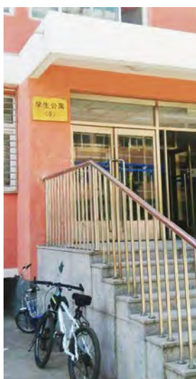
The student dormitory of Beijing University of Chemical Technology.
