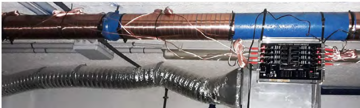
Step 2: Install the S250 unit on the water main
