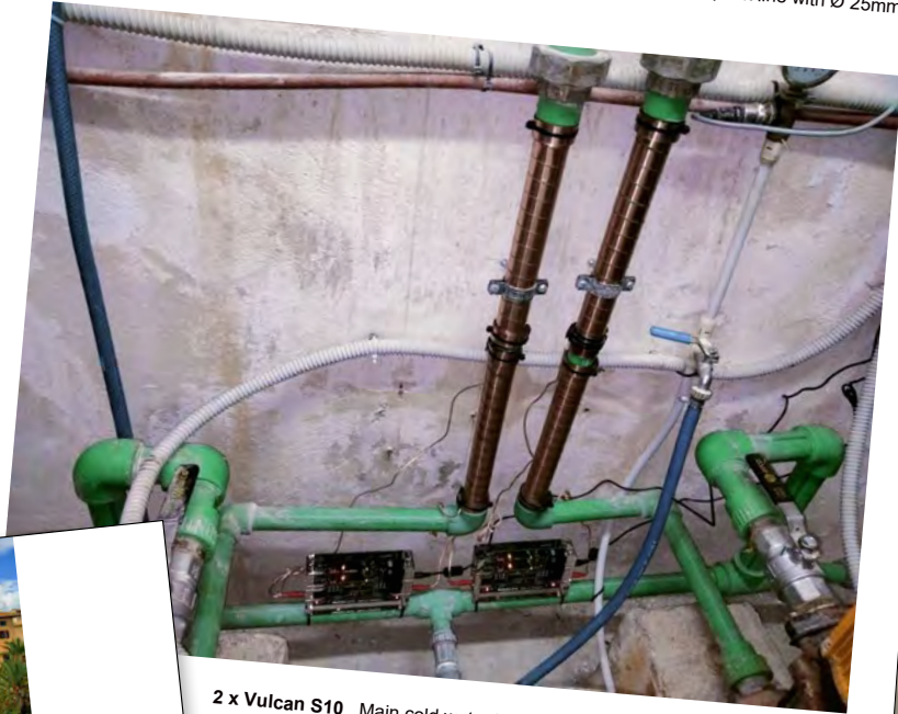
2 x Vulcan S10 Main cold water line with Ø 41 mm
