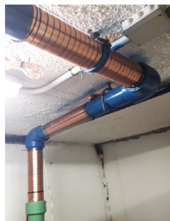
Schritt 1: Impulsbandinstallation
