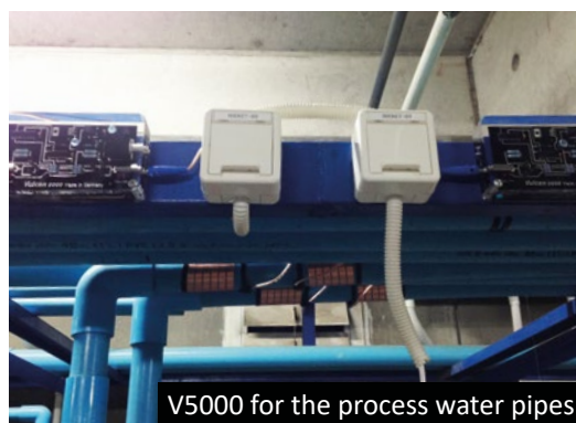
Impulse bands covered by pipe insulation
