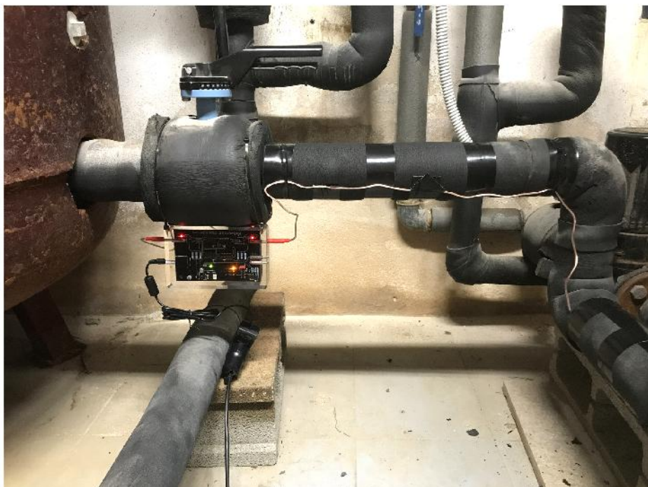
Vulcan S10 in the hot water circuit with Ø 63 mm
