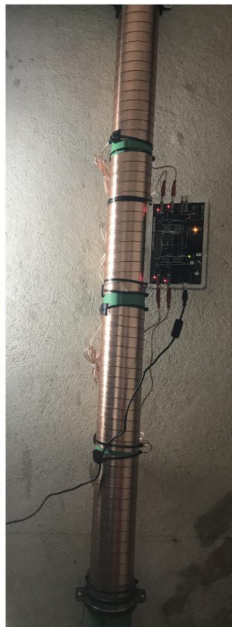
Vulcan S50 at the main cold water pipe Ø 90 mm
