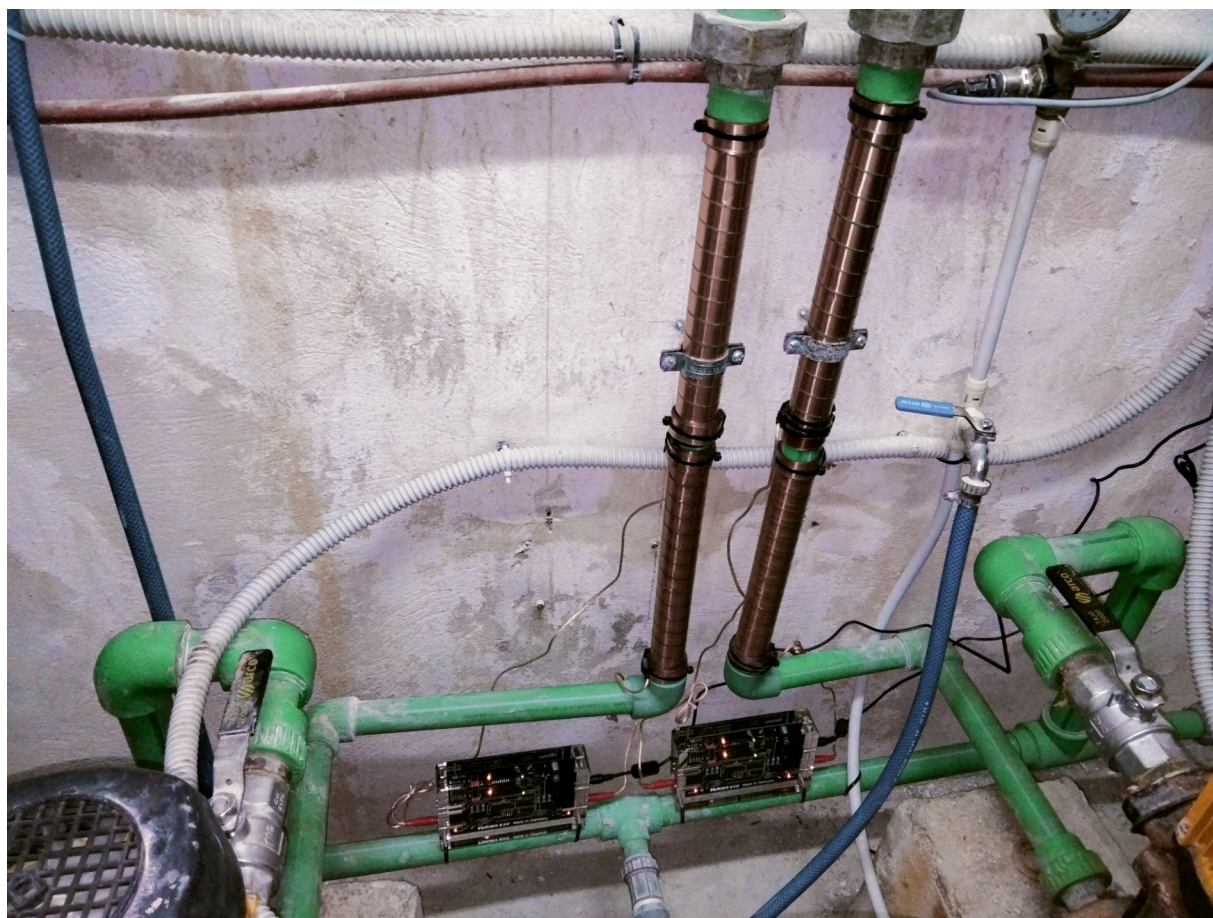
2 x Vulcan S10 Main cold water line with Ø 41 mm
